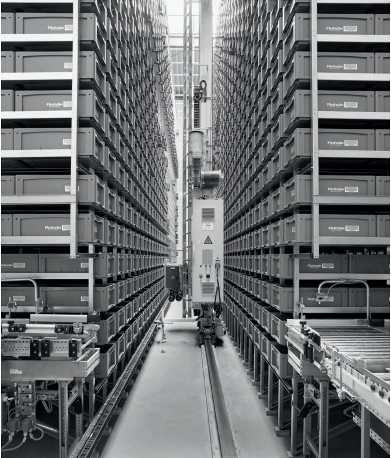
Werkbild: Rohde Automatisches Hochregallager Picture made by: Rohde Automatic high-bay warehouse
